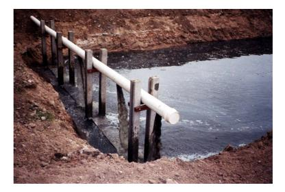
Solids-liquid separation and anaerobic degradation of septage in primary pond; the effluent is cotreated with municipal wastewater in a facultative (secondary) pond; settled solids are sun-dried and subsequently used in agriculture (Alcorta, Prov. of Rosario, Argentina)
